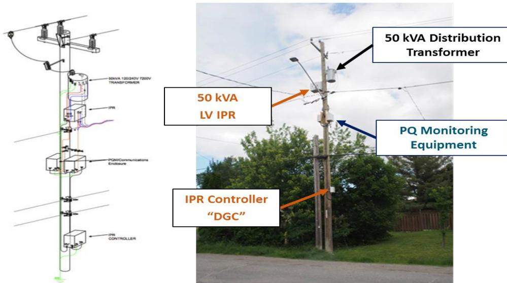
**Figure 7.** This drawing shows the planned configuration of the in-line power regulator (IPR) and controller with the distribution transformer and communications lines shown (left). In the final installation (photo, right), site-specific adjustments were made and the IPR was mounted on the opposite side of the pole from the transformer.
